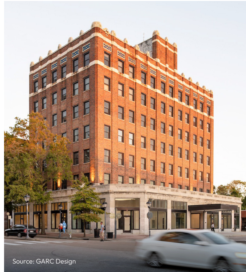
Figure 14 505 Washington Street - Professional Building
