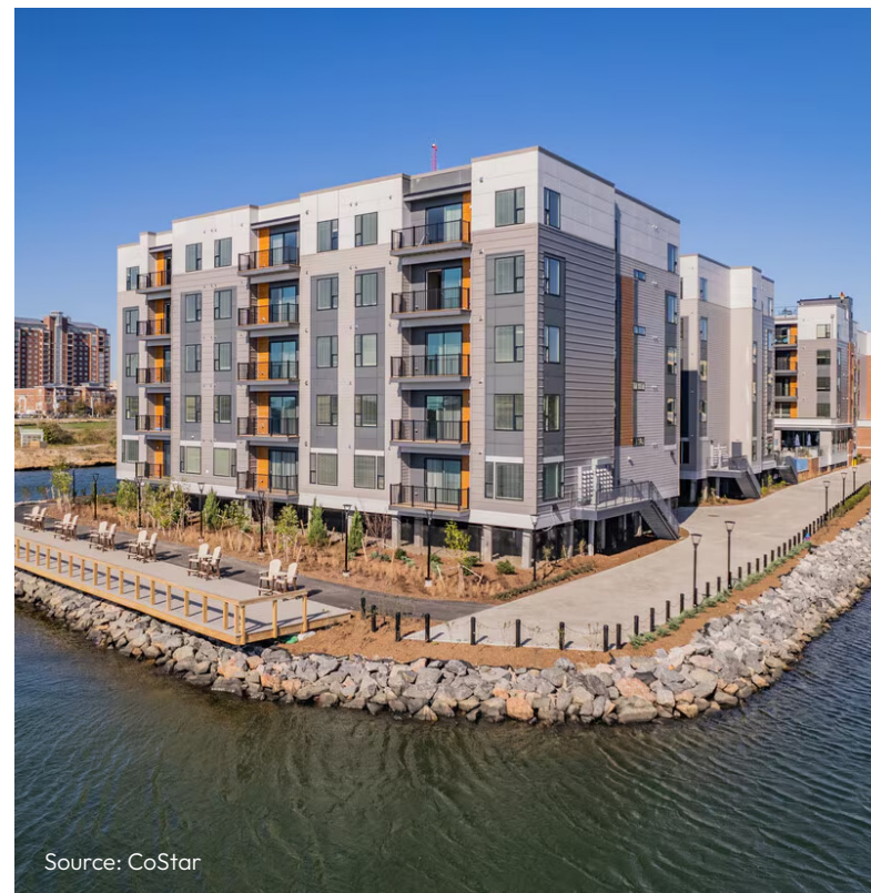
Figure 15 Lofts at Front Street
